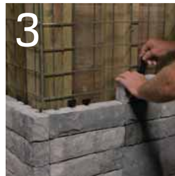
3 Attach Tandem Wall with Connector
