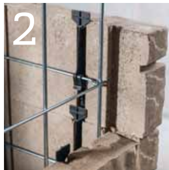
2 Use connector to attach veneers to grid
